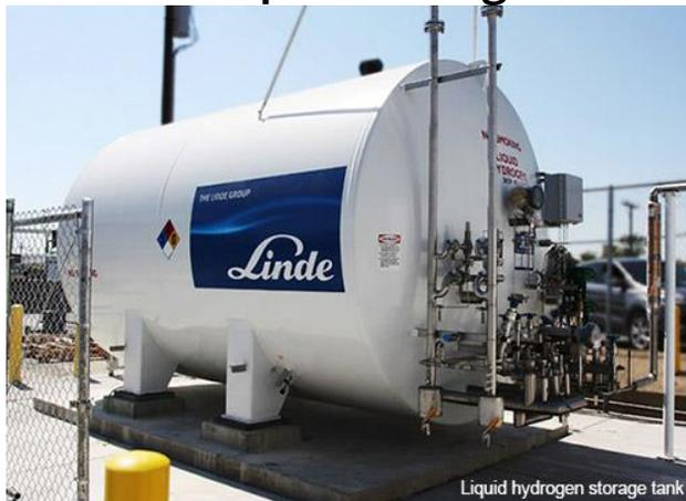
Liquid hydrogen storage tank
